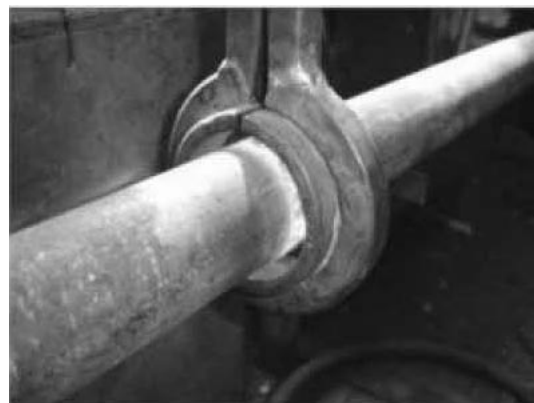
Fig. 3. Induction coil around the pipe during the welding operation.
