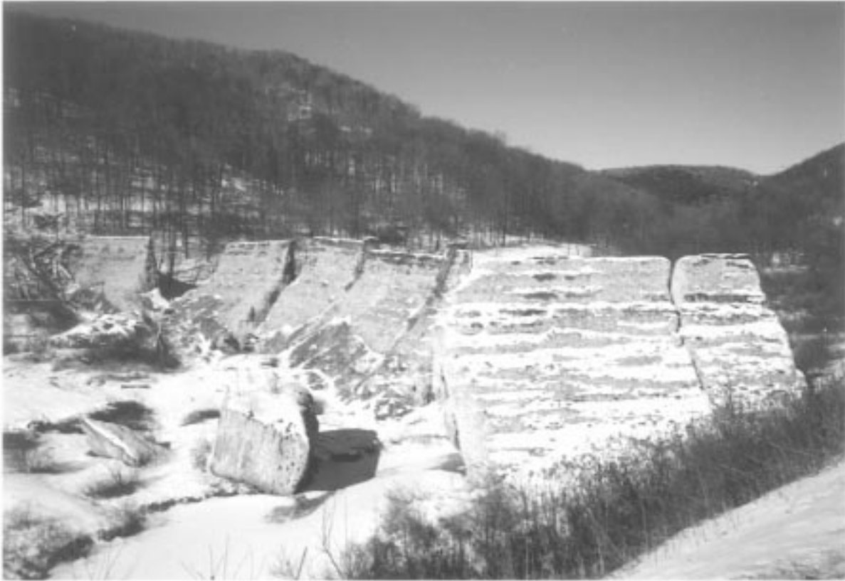
Fig. 2. The broken Austin Dam circa 2000.
