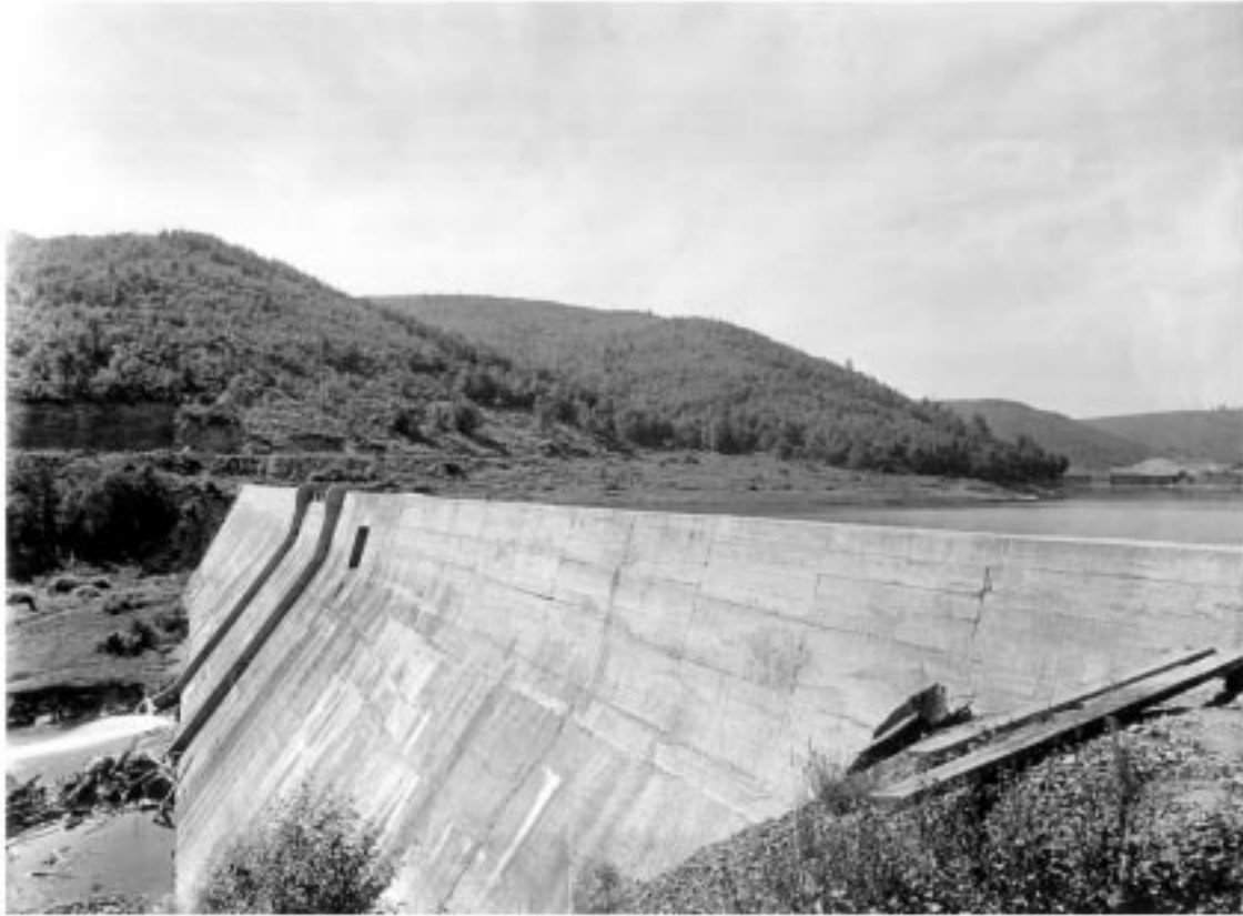
Fig. 1. The Austin Dam (courtesy of the Potter County Historical Society).
