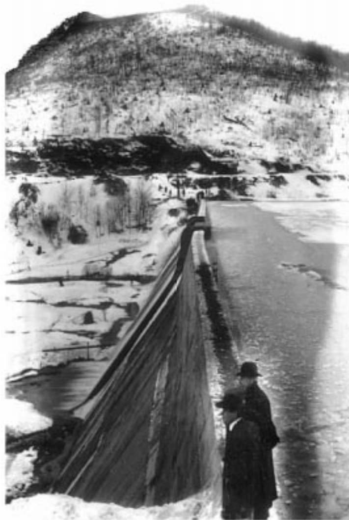
Fig. 6. The bow in the Austin Dam in the winter of 1910 (courtesy of the Potter County Historical Society).
